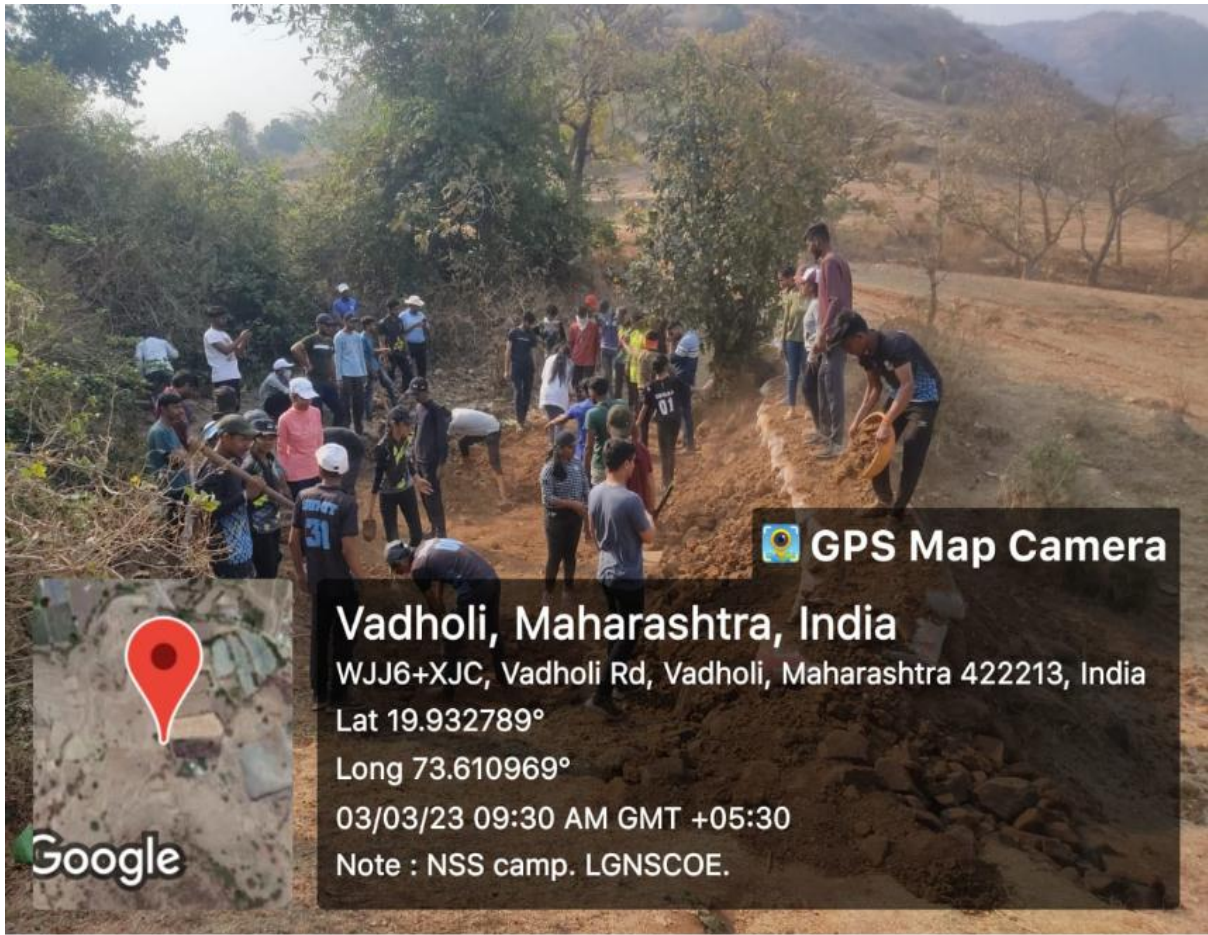
Dam Construction at Wadholi village during camp
