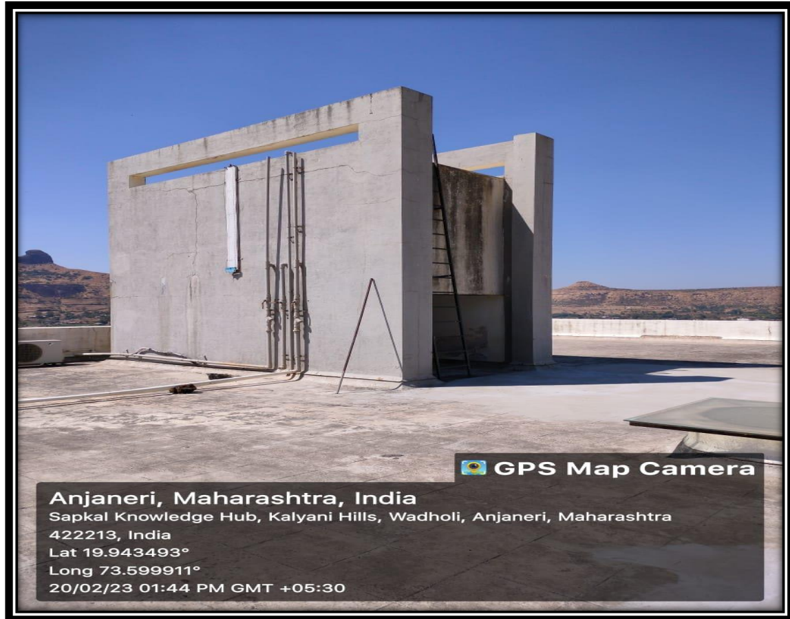
Overhead tanks & distribution system
