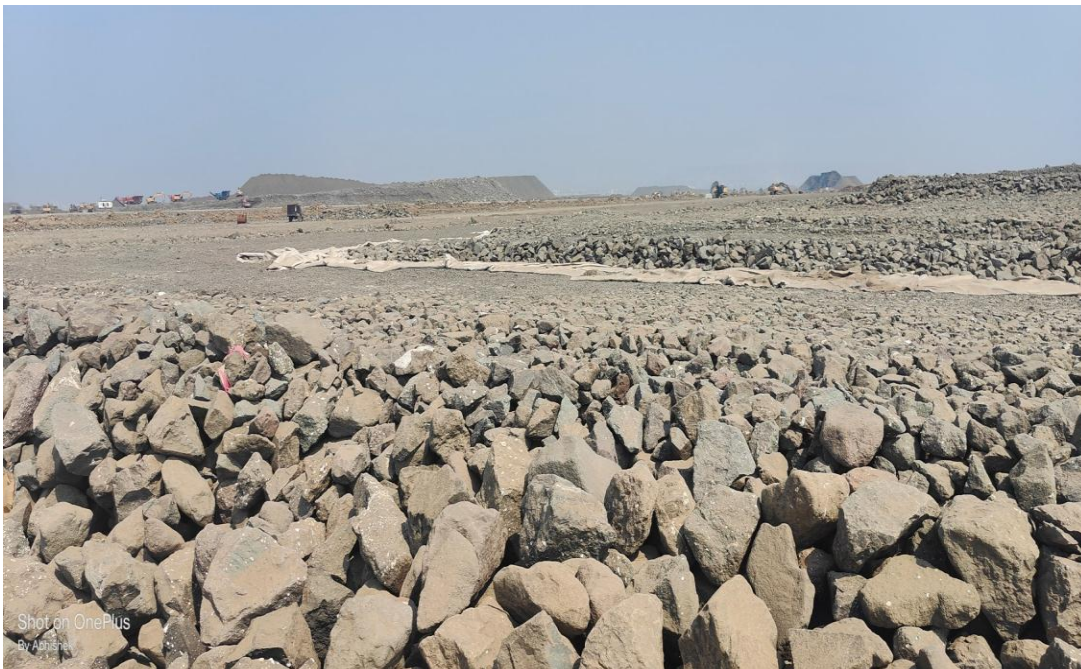
Figure 10: Local material used in the construction of the runway
