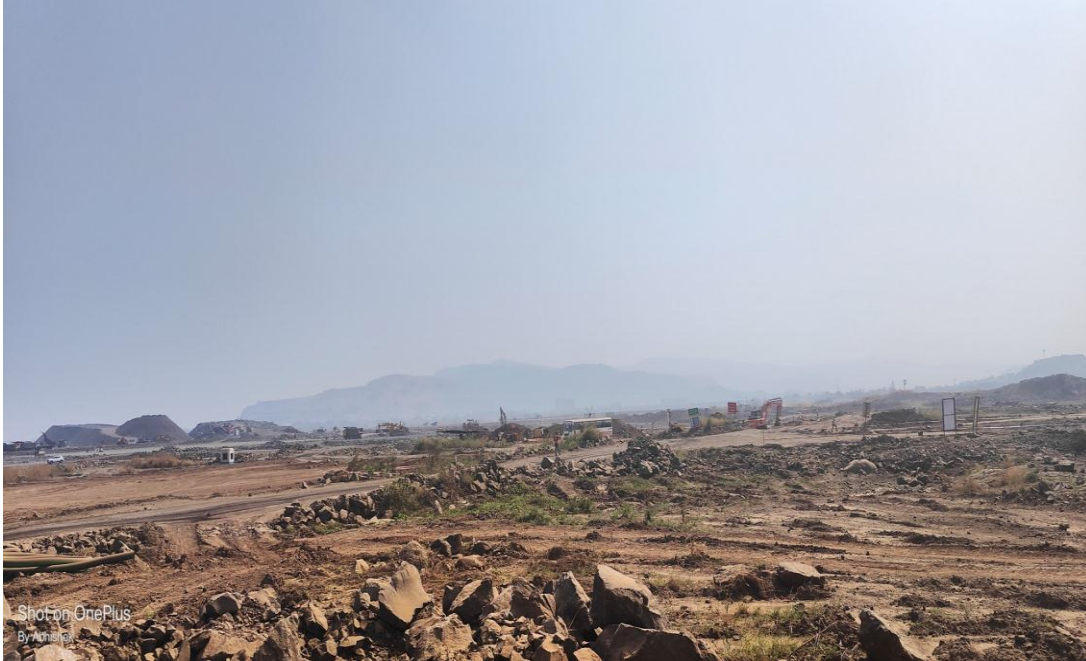
Figure 7: Runway Site before clearing the ground
