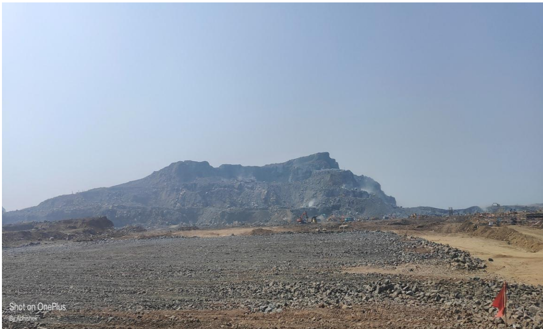
Figure 8: Runway site after clearing the ground
