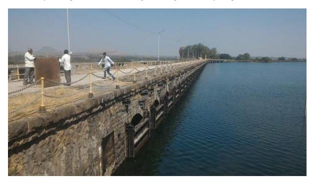
There are walls below the spillway of dam having huge floats of cylindrical shape. These floats are mechanically attached to the pulleys which are provided at the edges of all gates. These gates are operated on the counter base concept. When the float level is down, the gate gets opened as soon as when the well level rises the floats are lifted up, which leads to closure of gates. In this way discharge of water is allowed to pass through in Reynolds gates.
