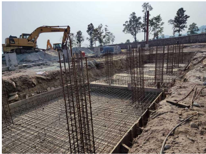
Figure 2 Detailing of Reinforcement
