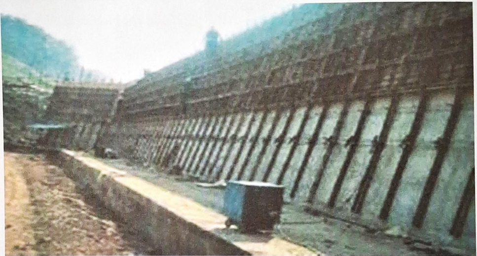
Fig. 4.6.2 RCC Retaining Wall Final stage
