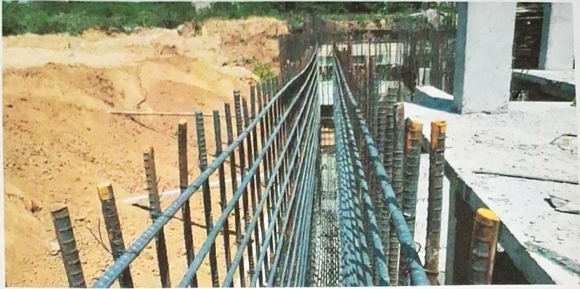
Fig. 4.6.1 RCC Retaining Wall Initial stage
