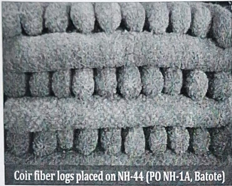
Old Coir fiber logs placed on NH-44 (PO NH-1A, Batote)
