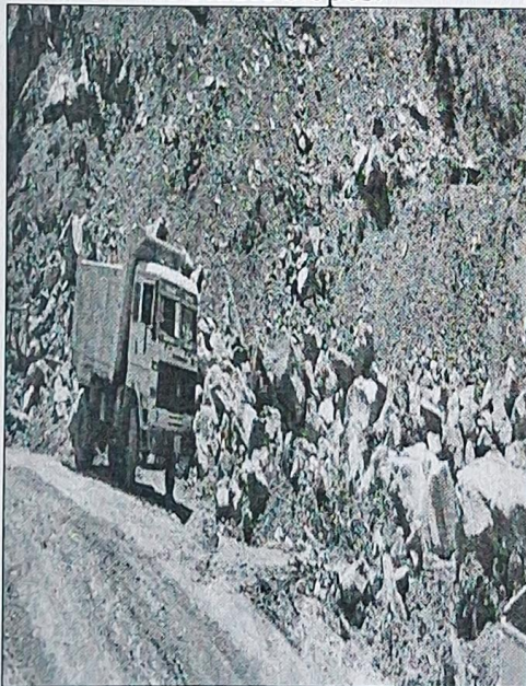
Rock Slope Collapse at Co. 70/Udh. Kheri
