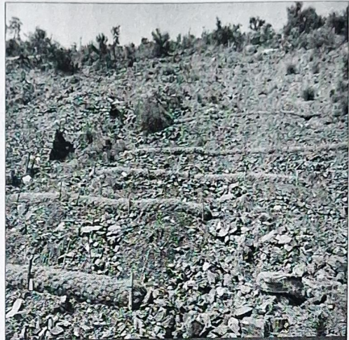
Coir fiber logs placed on NH-44 near Chenani-Nashri Tunnel
