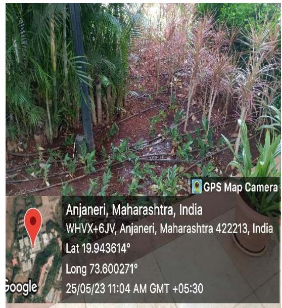
Geotagged photo of Drip irrigation system for plantation in the campus
