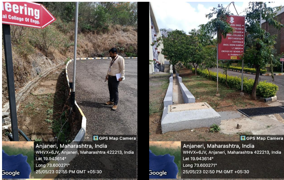
Geotagged photo of bunds constructed in the campus
