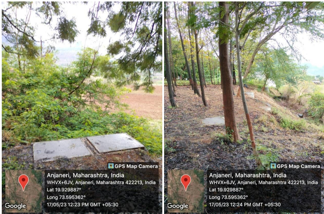
Geotagged photo of septic tank constructed by the institute
