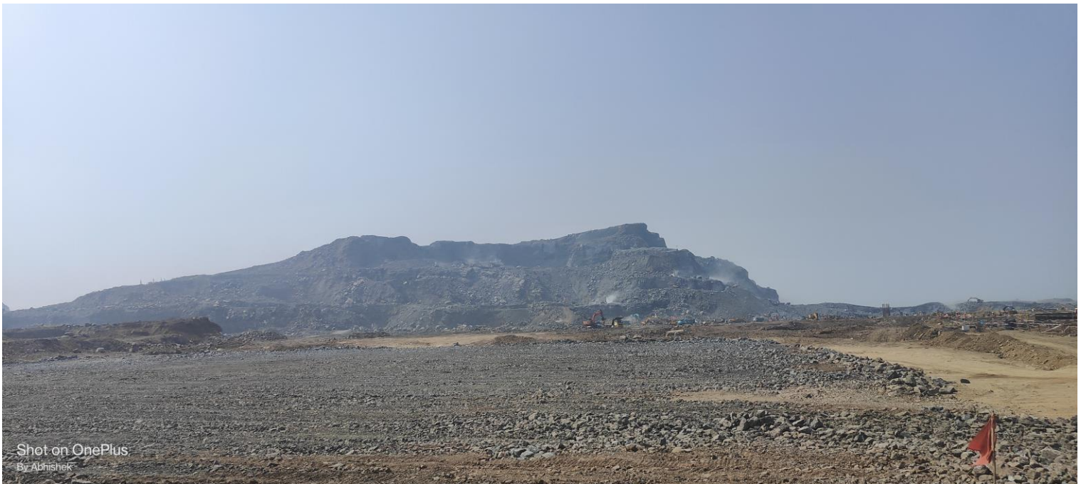
Figure 10: Runway site after clearing the ground
