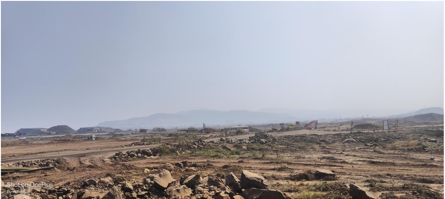
Figure 9: Runway Site before clearing the ground
