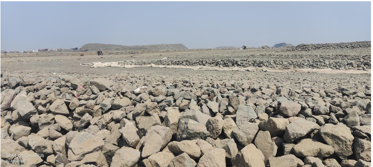
Figure 12: Local material used in construction of runway
