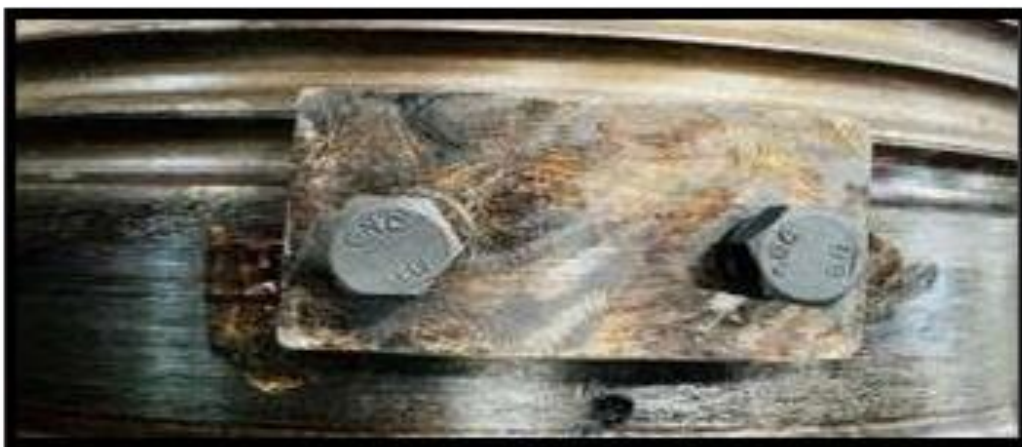
Figure 12: Drilling and bolted connection .
