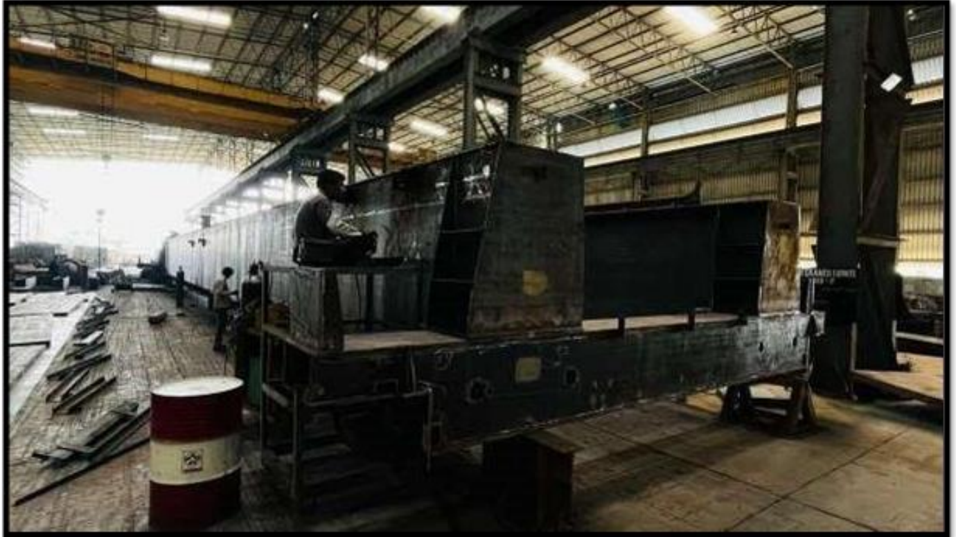
Figure 11: Students learnt the process of Design and Construction Gantry Girder
