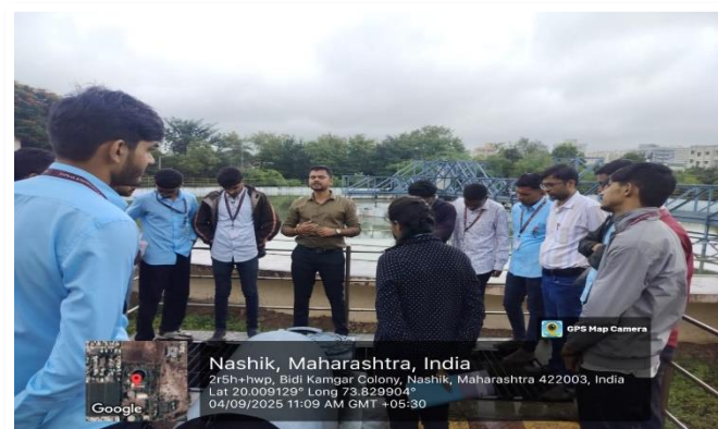
Visit to Nilgiri Water Treatment Plant, Nashik on 4 Sept 2025
